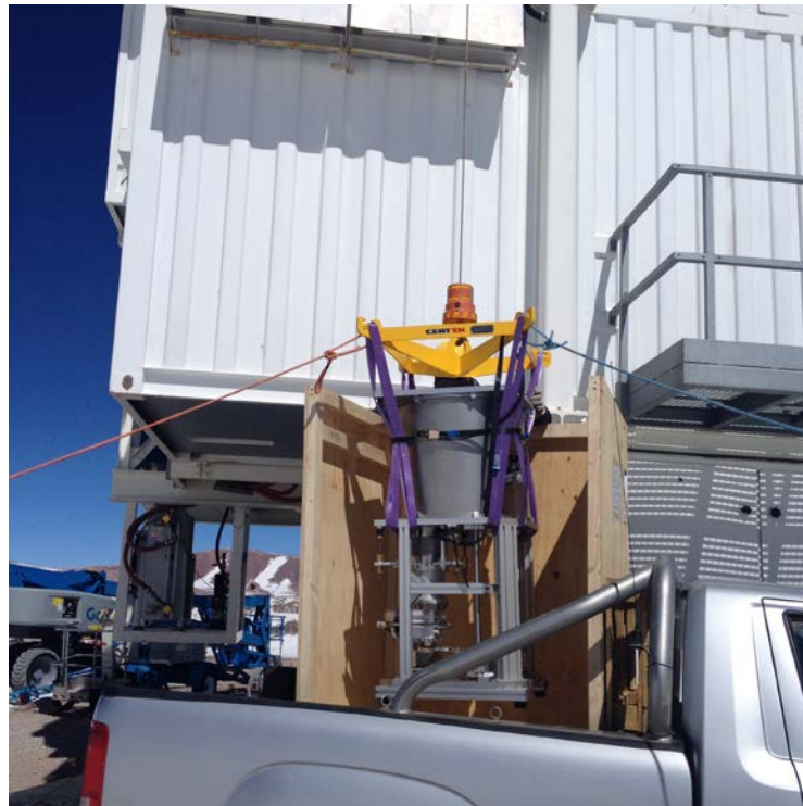
Lift of Sepia 2018-08-09. Note the yellow lifting device to which 4 purple straps are attached.
